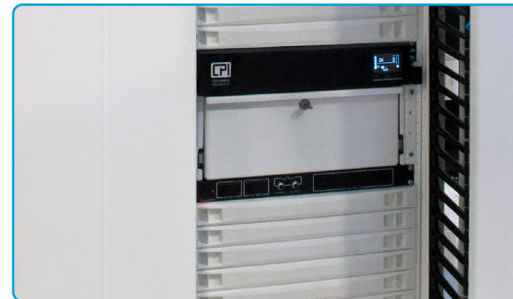
UPS Instalado
