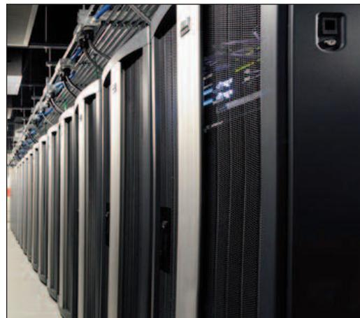
*CDW has installed 103 F-Series TeraFrame Cabinets with Vertical Exhaust Ducts in the first phase of their new data center.*
