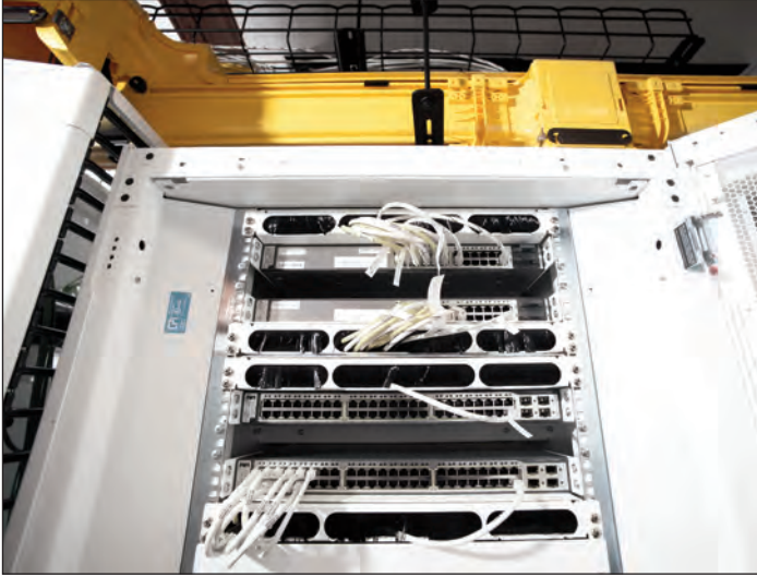
CPI Custom Air Box designed specifically for switches that require side airflow
