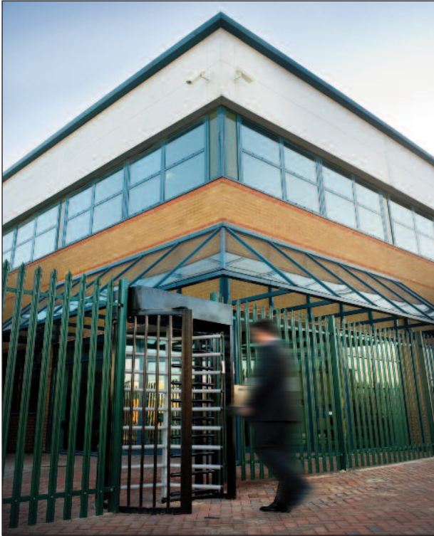
Powergate, TelecityGroup's eighth London data centre is at the forefront of data centre innovation offering colocation facilities with up to 20kW power per cabinet.
