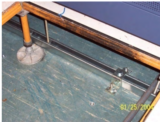
Fig. 2.3.2 Subfloor bracing
