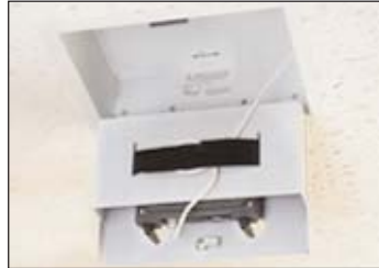
Installation of Access Points in ceiling mounted wireless ceiling enclosure and dome-style enclosure
