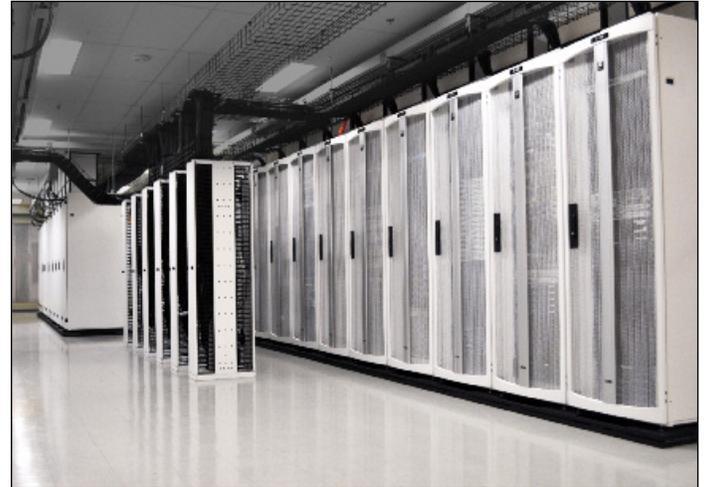
TCS built a showcase data center that earned two ASHRAE awards and a regular PUE of 1.15 by using 50 F-Series TeraFrame Cabinets with Vertical Exhaust Ducts, Evolution Cable Management and CPI Rack Systems.
