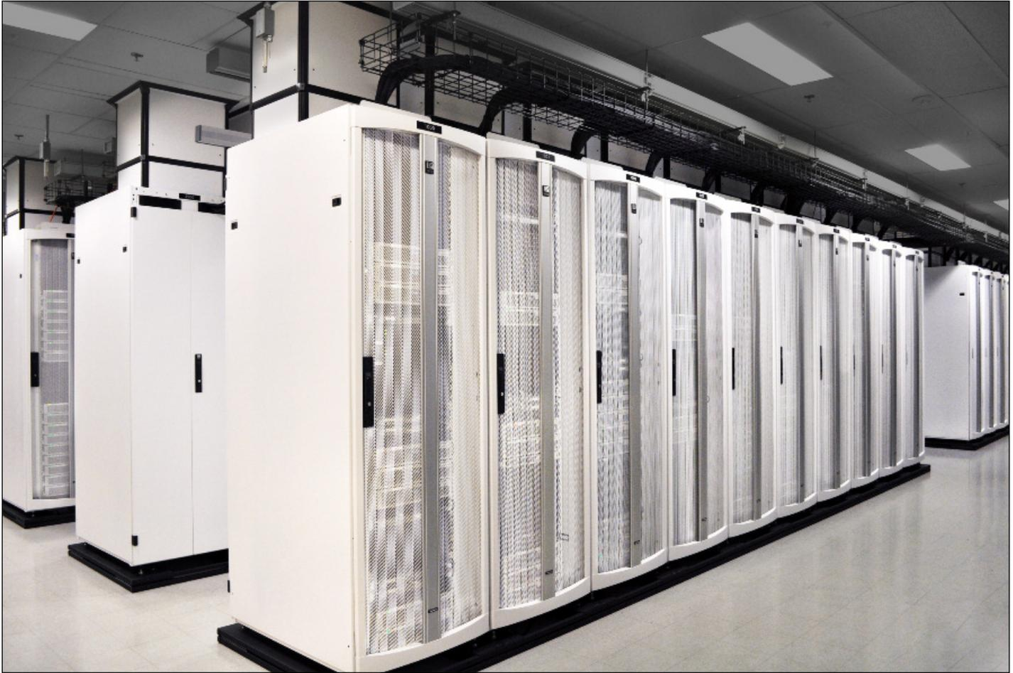
By containing the air and directing it into the ceiling through a Vertical Exhaust Duct, CPI's F-Series TeraFrame Cabinets helped TCS expand its data center with a cooling strategy that eliminated mechanical cooling and greatly reduced energy consumption.
