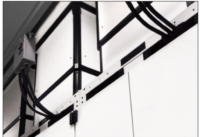
One of the ways TCS was able to optimize its cooling system was by keeping hot air contained in the cabinet and separate from the room through a combination of Vertical Exhaust Ducts and custom designed brush-sealed grommets.
