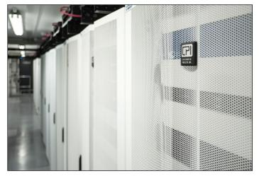
78 percent perforated doors on CPI's GF-Series GlobalFrame Cabinets maximize airflow.
