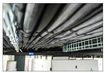
Even installed upside down to fit in the limited space, CPI's Cable Trays provide proper support to cables
