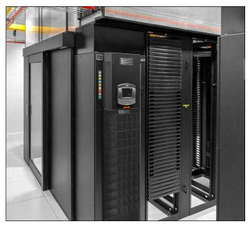
Evolution® Cable Management, Four-Post QuadraRacks, Aisle Containment Door Systems and Brushed Grommets were used to build a flexible solution that could be assembled on site.
