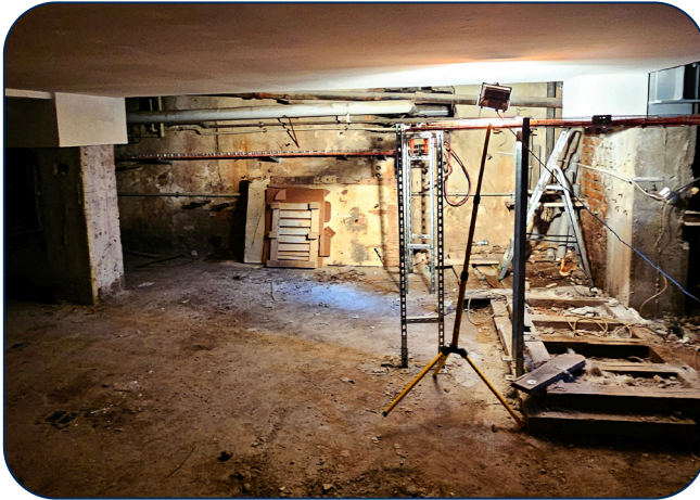
Bielański Hospital basement prior to construction
