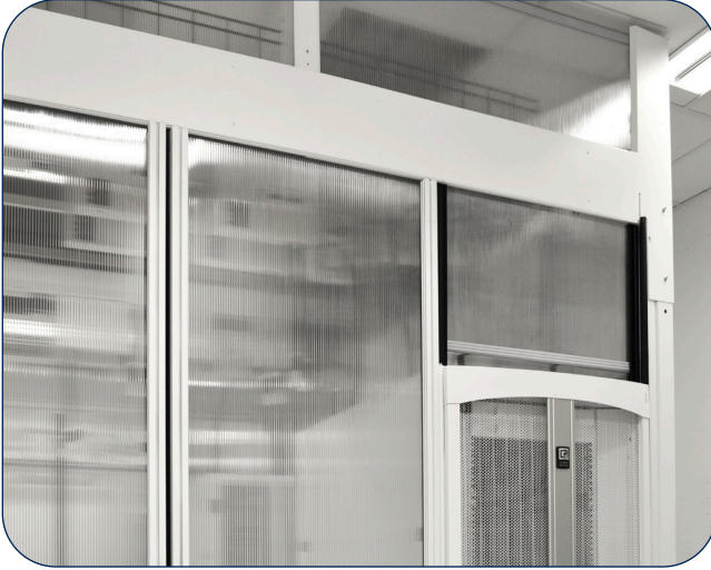
UF Health Shands utilized CPI's custom HAC Solution to maintain cooling, while accommodating storage solutions of various heights, widths and depths.
