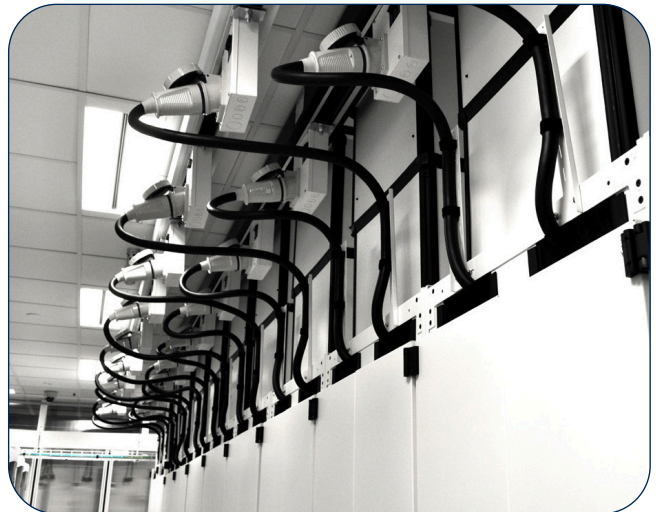
CPI manufactured custom cable openings into the cabinets to fit UF Health Shands’ unique design.
