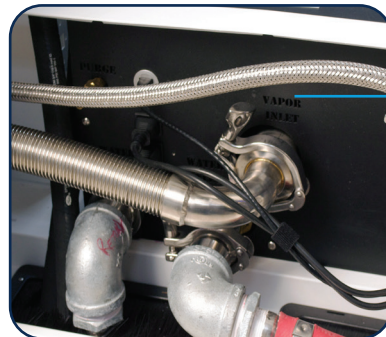
3 ZutaCore HyperCool Heat Rejection Unit (HRU-Water): A self-contained system placed inside 19" cabinet which can manage compute densities up to 100 kW total thermal load
