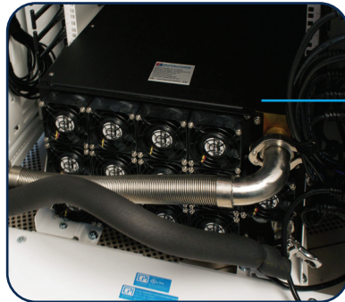
3 ZutaCore HyperCool Heat Rejection Unit (HRU-Air): A self-contained system placed inside 19" cabinet which can manage compute densities up to 20 kW total thermal load.
