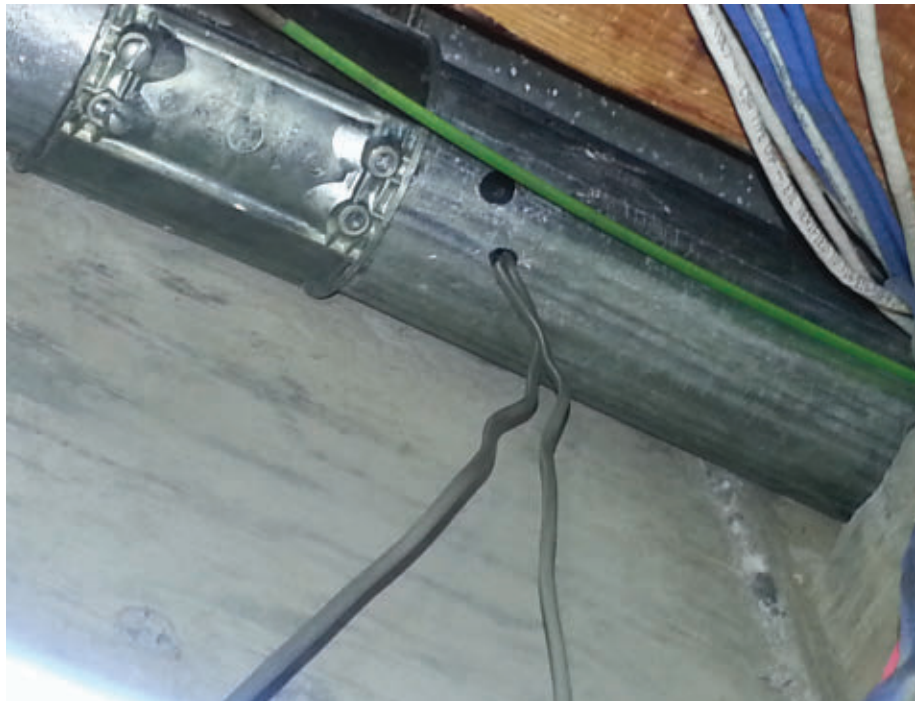
Drilled the conduit!
