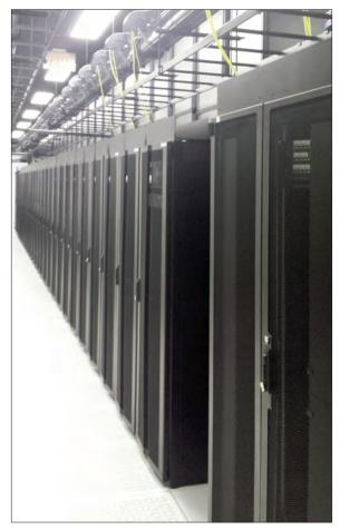
$\mbox{CPI}'\mbox{s}$  GF-Series GlobalFrame Cabinets with Vertical Exhaust Ducts were a part of the total Cologix solution (Vancouver site).
