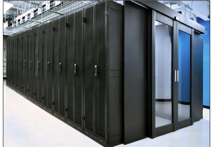
The doors of the CAC were a critical component to pressurize and seal the environment.
