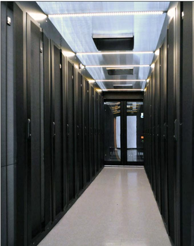
CAC was less expensive for Hostirian to build since they have the slab floor and no plenum.
