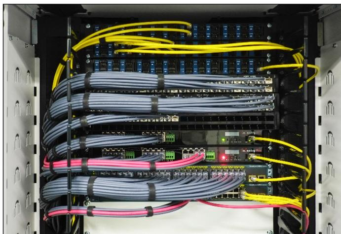
CPI's Finger Cable Manager accessory and Vertical Cable Manager with T-shaped cable guides have cable openings that align with each U space for patch cord management.
