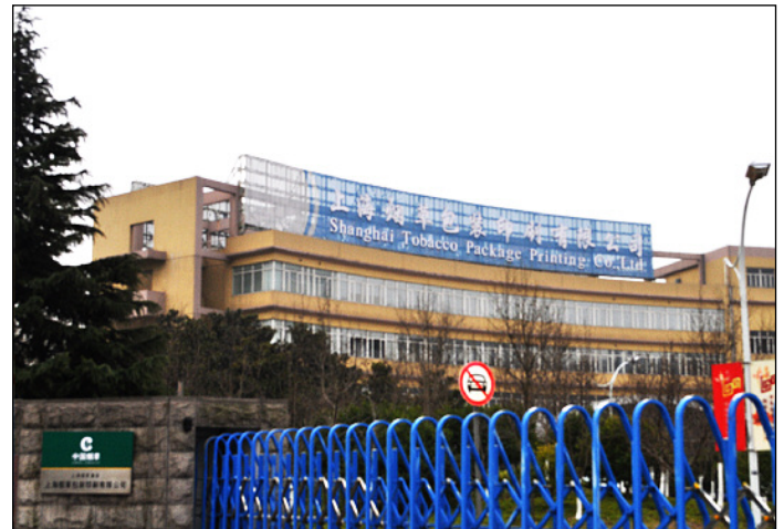
Shanghai Tobacco, China’s largest manufacturer of tobacco products, designed its disaster recovery data center as a model for efficiency. This need is especially critical in China, where a growing number of companies are having to overcome power availability issues on a daily basis.
