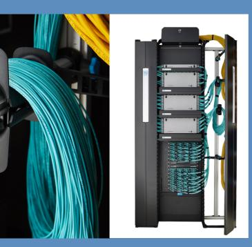
and connectors from any damage that can occur during routing or from hanging cable weight in vertical managers, and at connection and cable entry/exit points. Vertical cable managers also keep cables neat and organised within racks and cabinets, where substantial numbers of cables converge and terminate at network equipment and patch panels. This improves overall aesthetics, prevents spaghetti cabling that can impede proper airflow in and around equipment, facilitates access to
