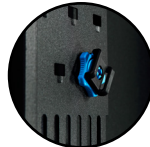
Cable Bundle Swivel, installed
