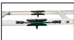
Ground Strap installed.
