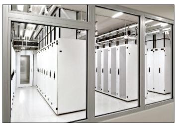
In an effort to build the greenest colocation facility in Oregon, the BendBroadband Vault deployed CPI Passive Cooling® and heat isolation by installing the F-Series TeraFrame® Cabinet System with Vertical Exhaust Ducts.
