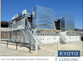
Two of the largest KyotoCooling® wheels in North America were installed at the Vault. Combined with CPI cabinets, they offer free cooling and a PUE as low as 1.2.
