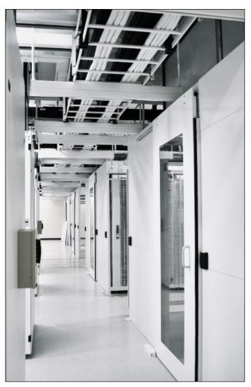
CPI used custom solutions such as white CPI Cable Runway and Cable Management to ensure the Vault's aesthetics would match those of a display facility with a high tech appearance.
