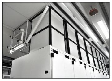
Vertical Exhaust Ducts direct heated return air into the plenum space, which isolates hot and cold air to create a containment solution that increases efficiency of both KyotoCooling® and traditional cooling systems.
